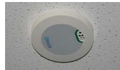
Left: Lighting control uses a MLS Pir detector in a DHL boardroom. right: MLS microwave detector, located in a ceiling tile.
